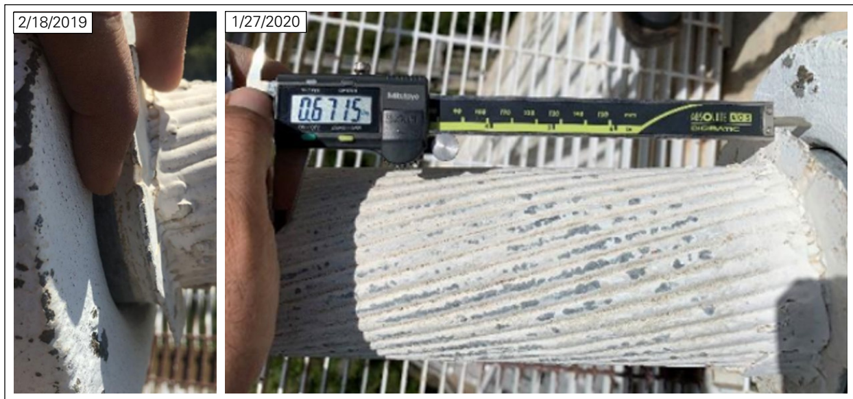
Figure 23: Cable slip at socket M12E_T (photos: NAIC Arecibo Observatory, a facility of the NSF).
