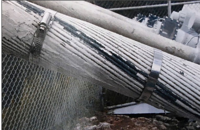
Figure 4: Original backstay B12-5 near anchor in 2003. Clamps and missing paint indicate a broken wire. Paint is also cracked between other wires ( photo: Ammann & Whitney 1 ).
