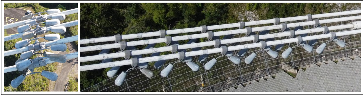
Figure 44: Stockbridge dampers near top (left) and bottom (right) of original M4 cables in 2020 (photos: NAIC Arecibo Observatory, a facility of the NSF).
