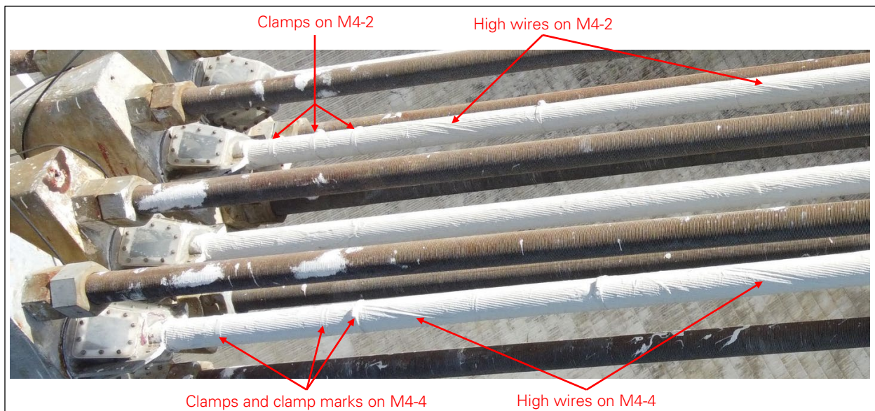
Figure 12: Evidence of past wire breaks at platform end of M4 cables (photo: NAIC Arecibo Observatory, a facility of the NSF).
