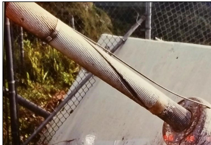
Figure 10: Wire break at ground end on B4-1 discovered on December 12, 1996 (photo: NAIC Arecibo Observatory, a facility of the NSF).
