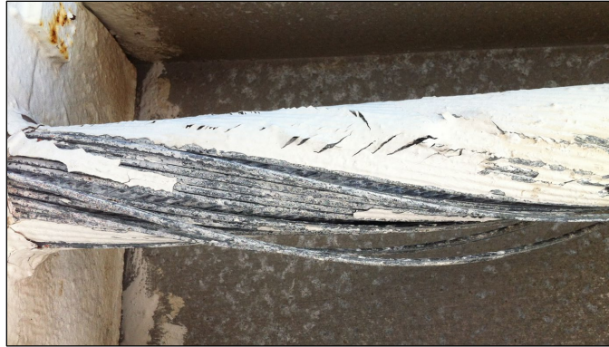
Figure 11: Multiple wire breaks near M8-4 splice discovered on January 14, 2014 (photo: NAIC Arecibo Observatory, a facility of the NSF).
