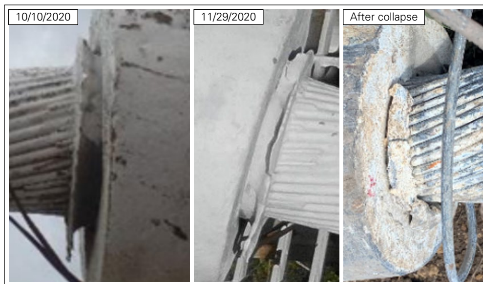
Figure 22: Cable slip at socket M8S_T (left photo: WJE 10 ; center photo: NAIC Arecibo Observatory, a facility of the NSF).
