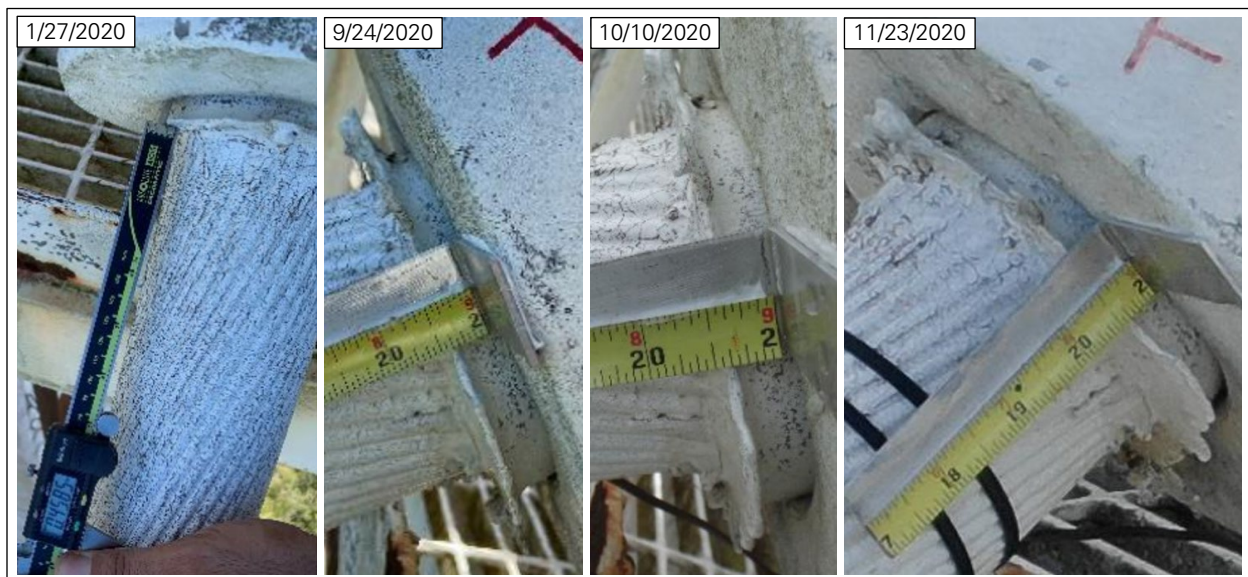
Figure 37: Cable slip at socket B12W_T (left and right photos: NAIC Arecibo Observatory, a facility of the NSF; center photos: WJE 14 ).
