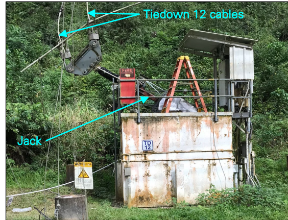
Figure 7: Base of tiedown 12, after telescope collapse.
