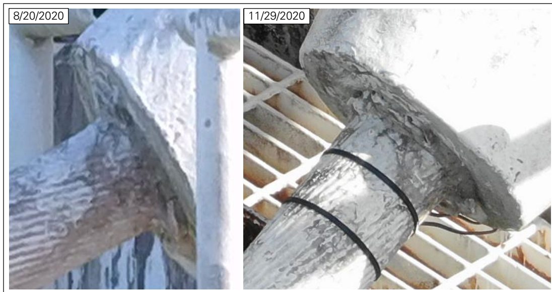
Figure 35: Cable slip at socket B8S_T (photos: NAIC Arecibo Observatory, a facility of the NSF).
